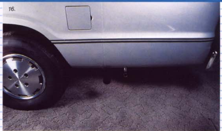
'Onan MicroLite' generator is vented through the floor so that no more than an exhaust pipe is visible from the outside.
